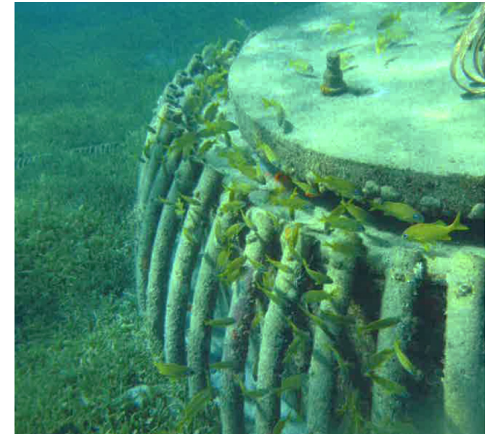
Eco-designed mooring with habitat for juveniles on the block (Pioch)
